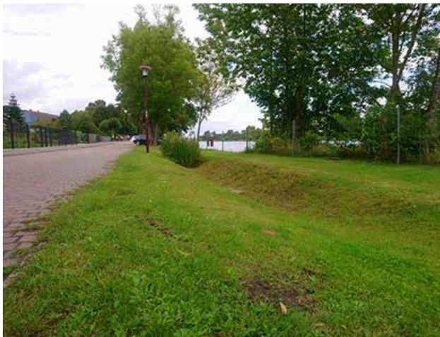
Fig 16: Bioswale next to a bike-path in Gartz, 2019
